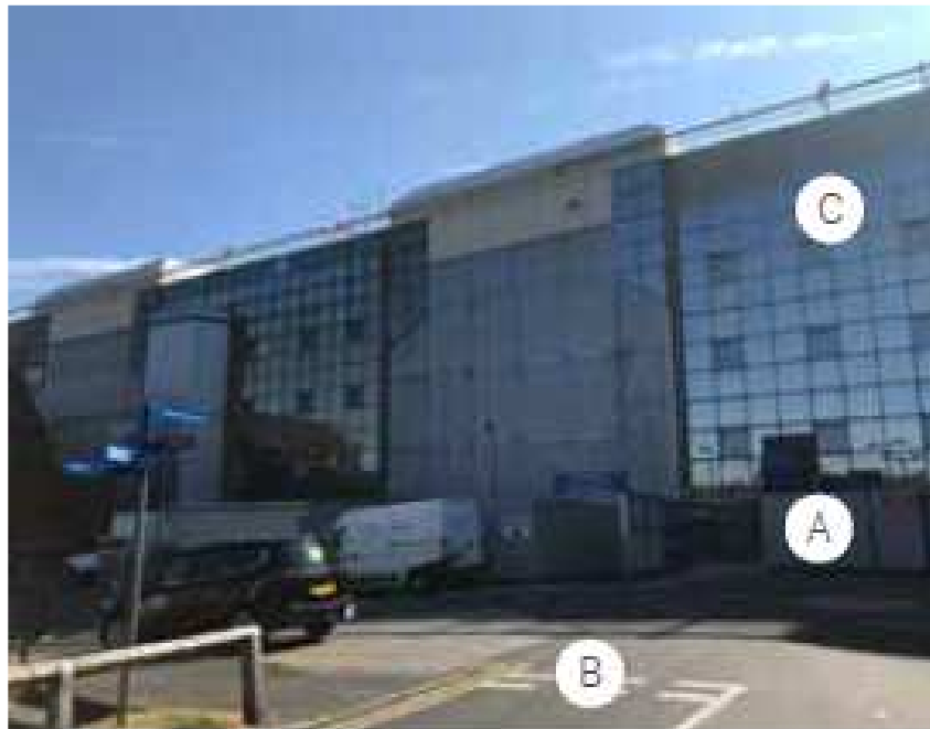
05. VIEW OF EXISTING HOSPITAL FACADE
